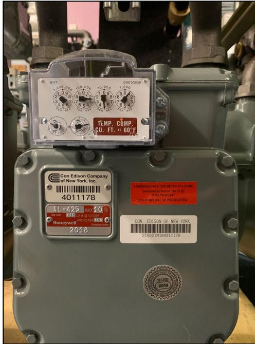
*Honeywell American Meter AC-250 Class Gas Meter*
